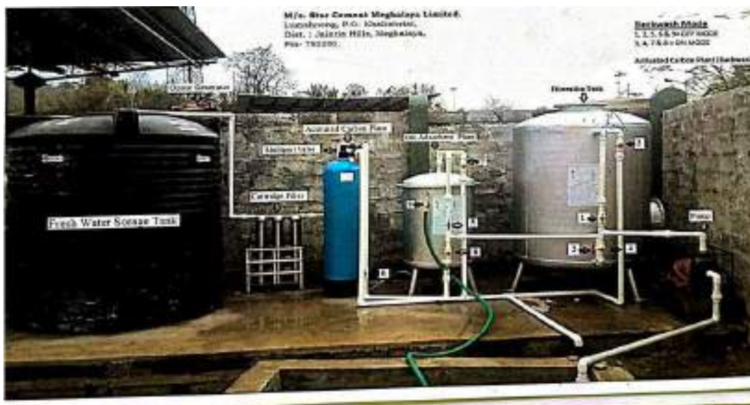
FIGURE-3 EFFLUENT TREATMENT PLANT OF 20 KLD
